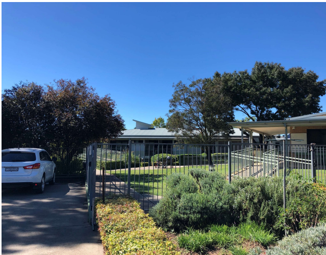
Image – Rear access from Queen Street
