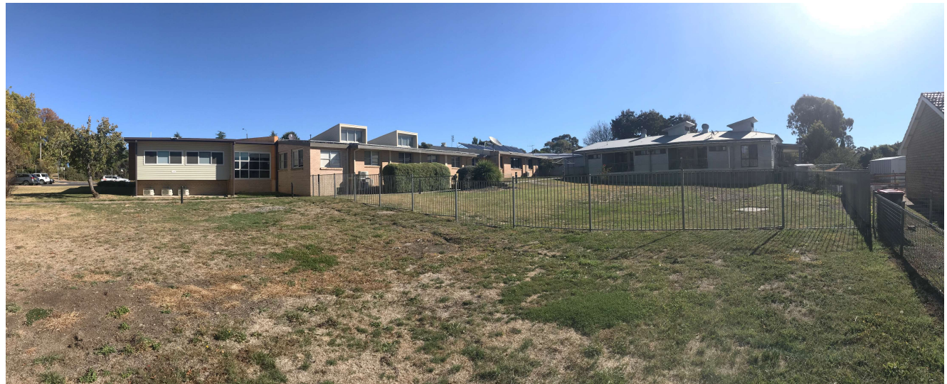
Figure : View of rear vacant zone behind the existing RAC buildings
