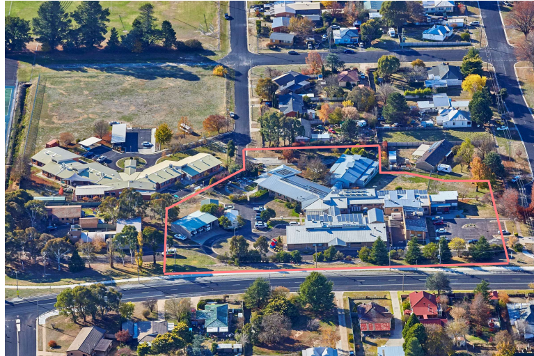
Image – Aerial view of the existing site
